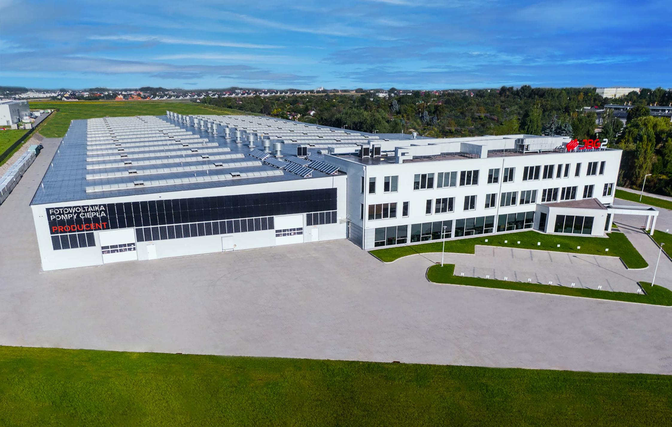
ŽORY MANUFACTURING PLANT
